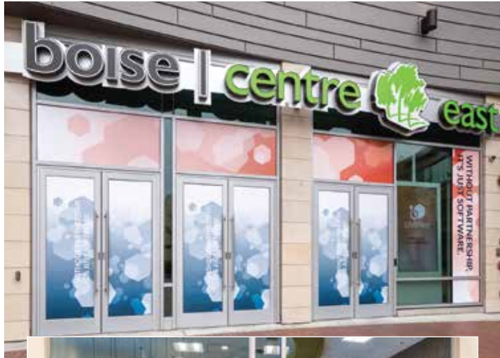
A Main Entry Doors, Vestibule Doors, and Side Panels off The Grove Plaza
