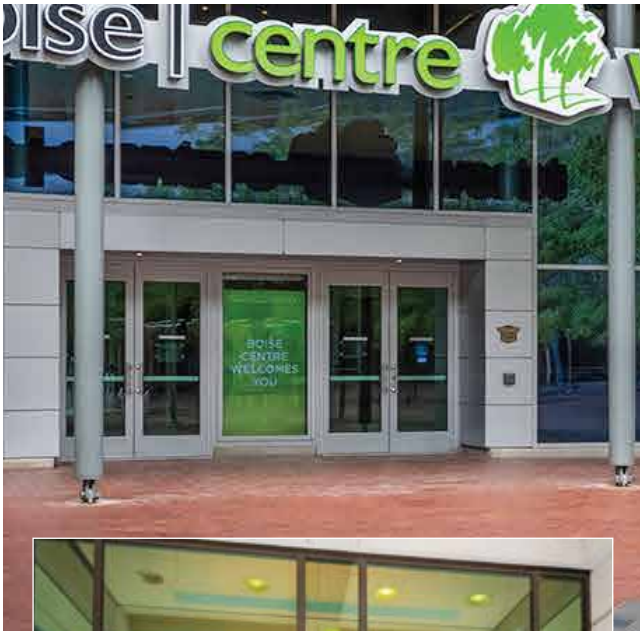
A Main Entry Doors, Vestibule Doors and Side Panels off The Grove Plaza
