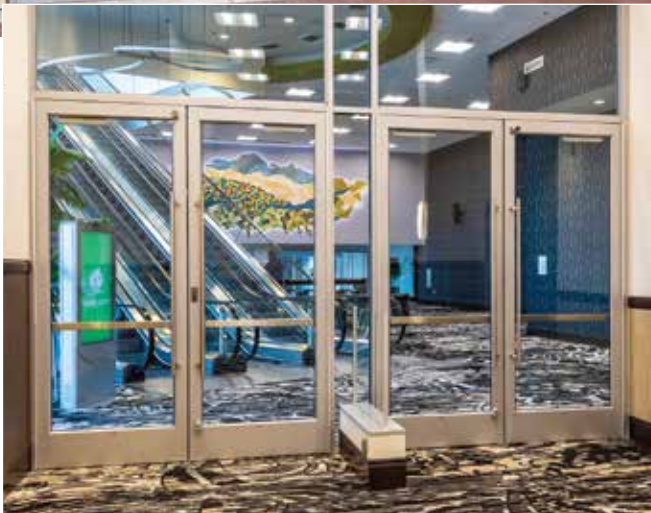
B Interior Entry Doors and Side Panels (2nd Level)
